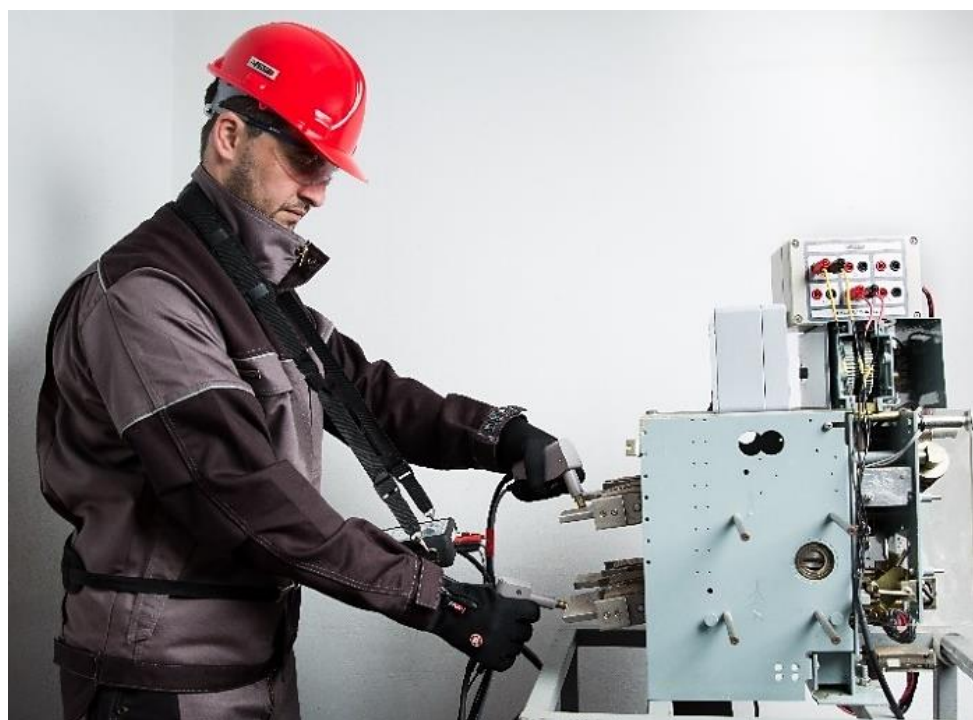
Figure 3-4: Connecting RMO-H to circuit breaker using cables with Kelvin probes
